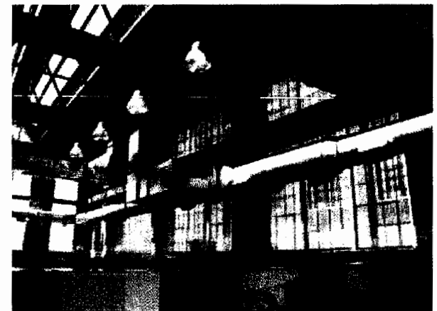
[5-6] Large windows and a roof monitor provide natural illumination in a historic industrial building.
