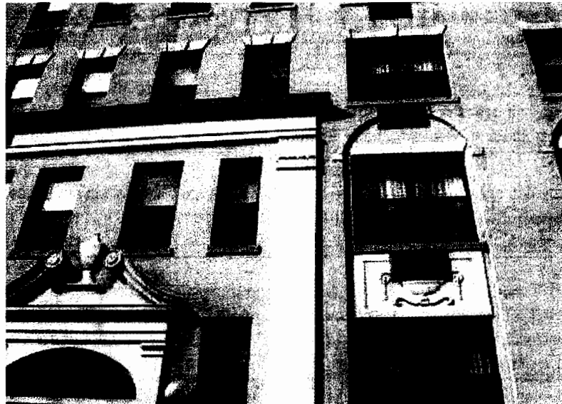
Not Recommended: [61] The cuts made in the brick and the decorative stone trim to install through-the-wall air conditioners have not only destroyed building material, but have also negatively impacted the character of this historic apartment building.
